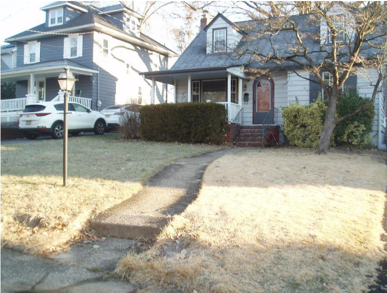
FRONT VIEW FROM SECOND AVENUE
