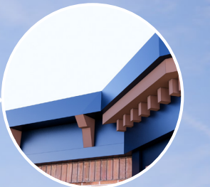
PAINTED POLY-ASH CORNICE & BRACKETS
