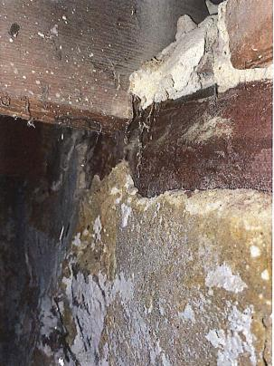
**Joist Deflection (Sagging).** The 1st floor joists are deflecting and causing the floor above it to sag. This deflection is the result of damage and/or overloading due to the installation of various mechanical and plumbing systems. As a result the structural integrity of the damaged joists have been compromised and will need to be reinforced.
