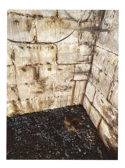
**Foundation Undermined.** Certain portions of the foundation for the building were undermined and are now unstable. Additionally the foundation for one of the main support columns was also undermined.
