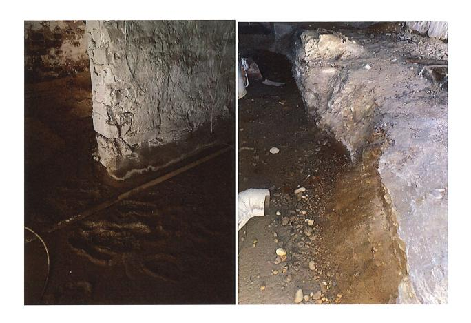
**Foundation Damage** There are large holes in the foundation wall. These holes are the result of the installation of various mechanical, electrical and plumbing systems. These holes greatly affect the integrity of the foundation.
