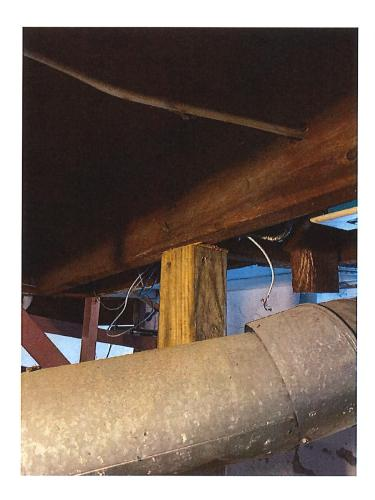
**Joists Bearing Failure.** The joists on the sides of the basement are compressing where they rest on the exterior wall. This type of failure is called a bearing failure and is the result of water infiltration on the exterior wall that is damaging the joists and causing it to compress. As a result of this compression the floors above the joists are starting to deflect and sag.
