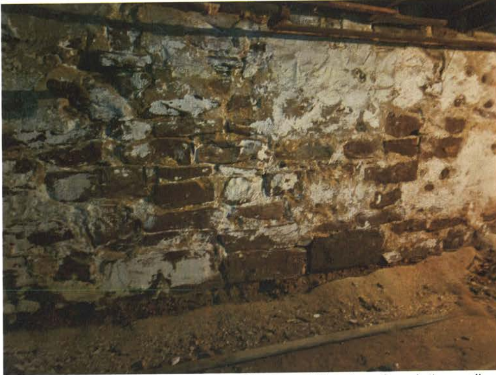
Photograph 6: Portion of exposed bottom of flagstone foundation wall
