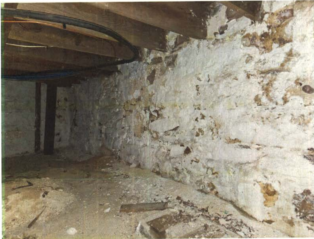
Photograph 5 : Flagstone foundation wall with original basement floor
