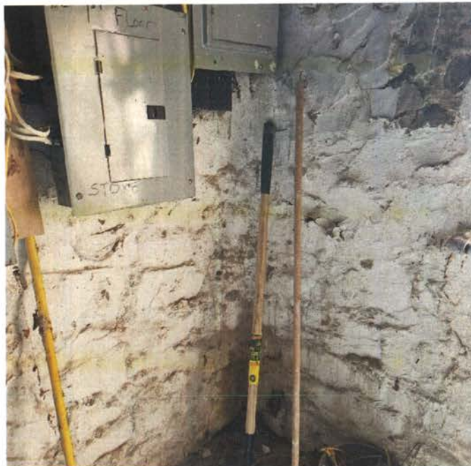
Photograph 4 : Flagstone foundation wall adjacent to bilco access
