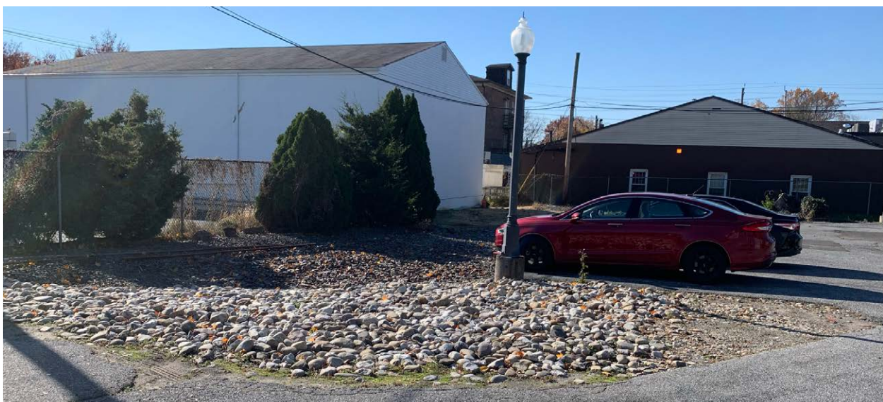
Figure 12. An individual site intervention contributing to off-site flooding issues on Block 25
