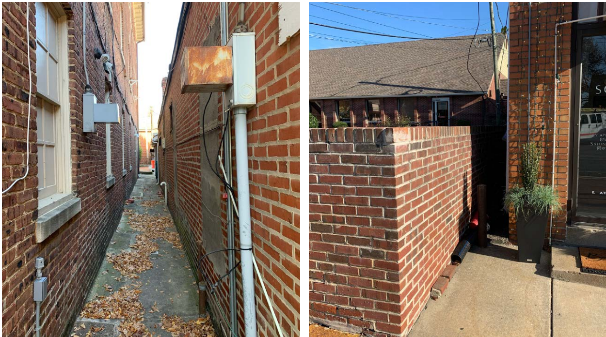
Figure 11. Excessive land coverage resulting in narrow alleyways, limiting access
