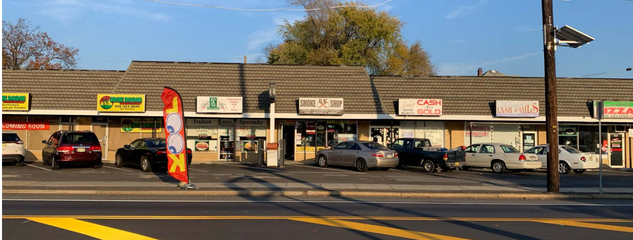
Figure 9. Mid-block parking access along Black Horse Pike
